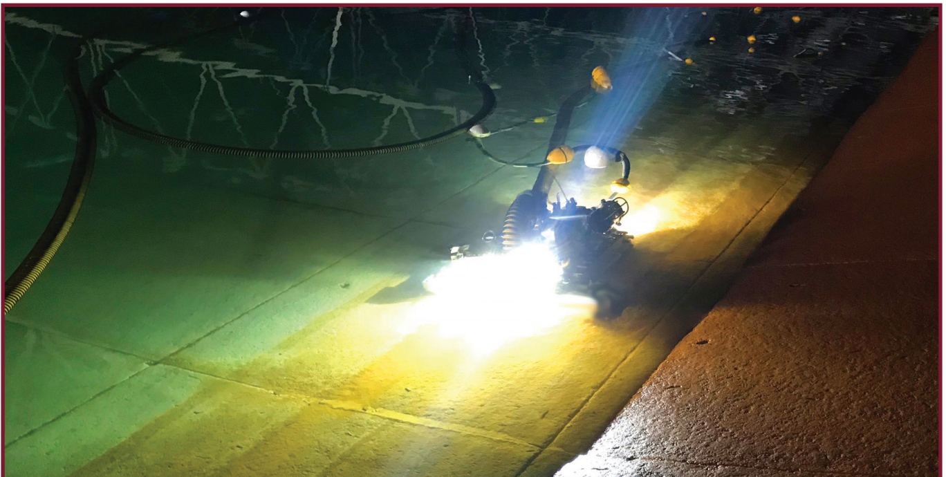
Potable tank cleaning robot removing sediment while the asset remains online.
