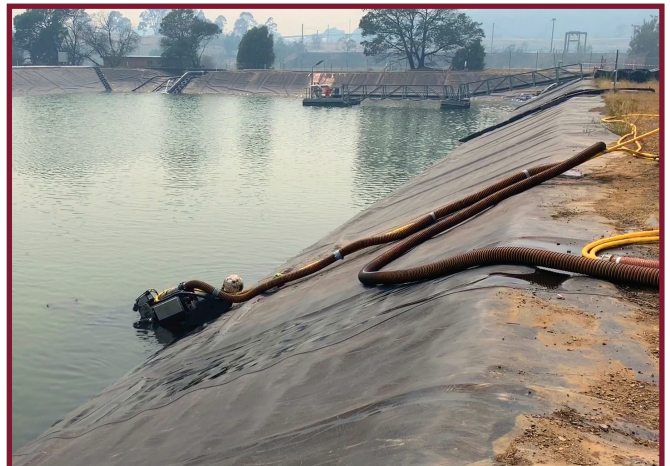
Liner-safe robot cleaning a HDPE lined process pond.
